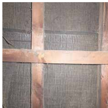
(xii) New roof timber/ felt
