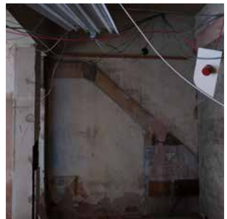
Evidence of past staircase (Ground Floor)
