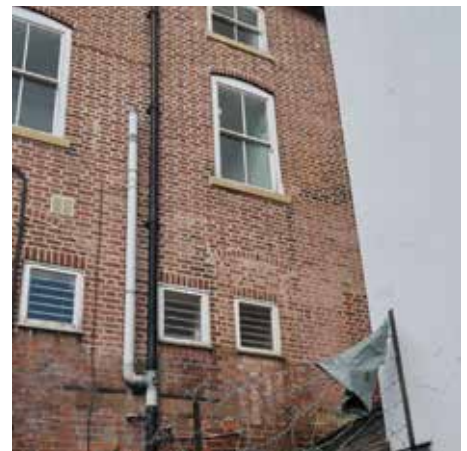
Evidence of previous openings
