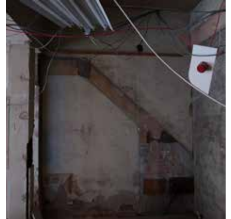
(ii) Evidence of lost stair (North)
